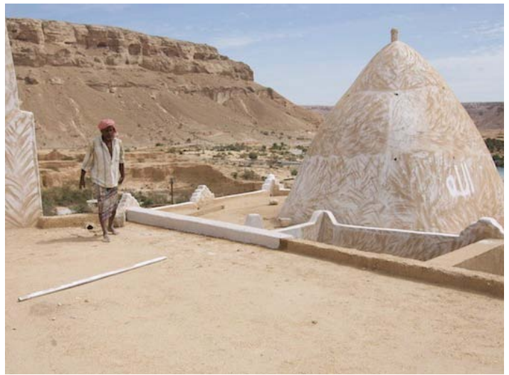
Photo: Sah Mosque under Construction © Salma Samar Damluji
